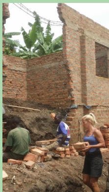
Rebuilding the walls at Solid Rock School
