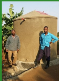
Ferro cement water tank
